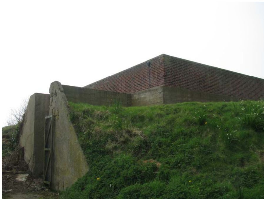
Fig 3 – Corner view of Receiver Block with Blast Wall
